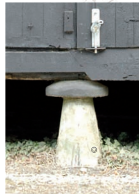
'Mushroom Stands' were designed to prevent rats and mice from jumping or climbing into a granary. Mushroom Stands can be seen at the Granary, Wall Hall
