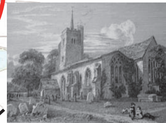
St John the Baptist site was first consecrated c960AD. The only Grade 1 listed building in the Parish of Aldenham.
