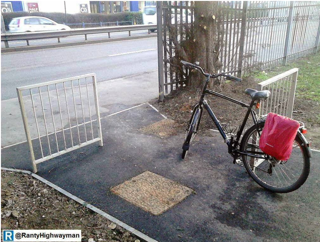
Metal barriers – Type G7 – two of these are proposed at the junction between Elm Walk footpath and the allotment track
